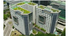
1. Building Integrated Photovoltaic, 건물일체형 태양광
